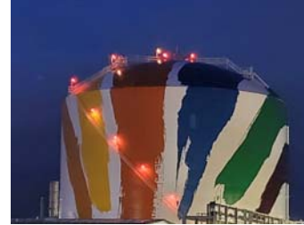
Photo: National Grid
