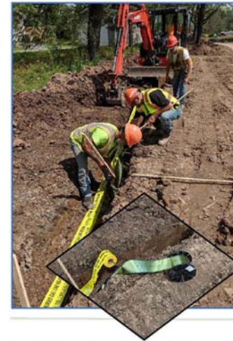
This photo illustrates field installations of MetGlas® in National Fuel Gas territory in Buffalo, NY in 2019 - part of a project to evaluate amorphous metal tape as a practical application for PE pipe location. Source: NYSEARCH
