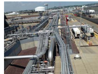
LNG delivery trucks fueling at the Everett LNG facility, for transport to a local gas distribution company facility.
