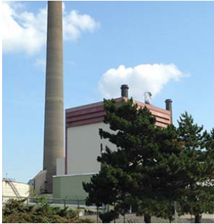
Natural gas power plant near Boston.
