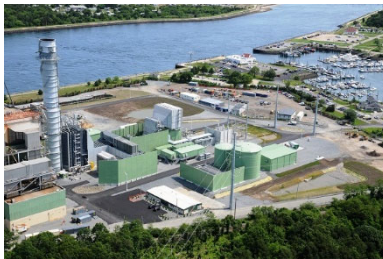
NRG Canal 3 Sandwich, MA 333 MWs Online June 2019
