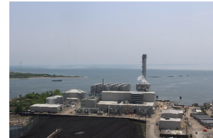
PSEG Power Bridgeport Harbor Station 5 Bridgeport, CT 485 MWs Online June 2019
