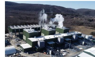
Cricket Valley Energy Dover, NY 1,100 MWs Online Spring 2020
