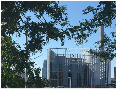
In 2020, Harvard’s new central energy facility in Allston, MA became fully operational. It runs primarily on natural gas.
