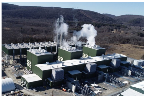
Photo: Cricket Valley Energy Center
