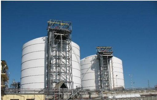
Everett LNG facility, part of Exelon (Constellation)
