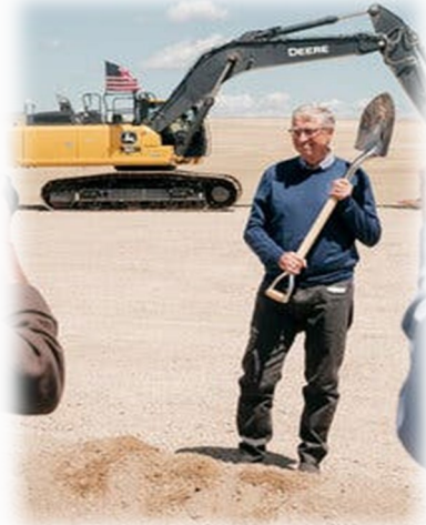
TerraPower Natrium – site preparations underway in Wyoming
