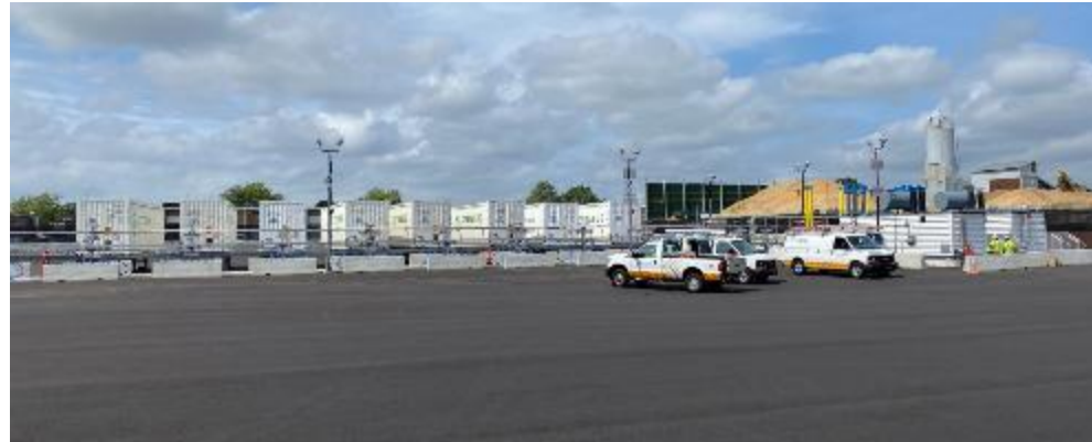
Compressed Gas Injection Station
