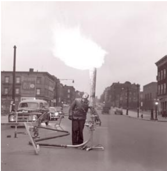
A purge burner igniting manufactured gas being replaced in a main by natural gas during the 'great conversion' in 1952
