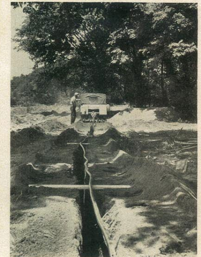
GROUND PIPE for heat pump is laid in deep trench dug by jeep-drawn ditch digger. Pipe is buried below frost line where year-round temperature remains nearly constant. Here in Jeffersonville, Indiana this temperature is about 52°F.
