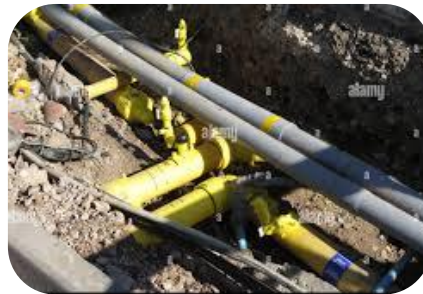
Repair/Replace Leak-Prone Pipe
