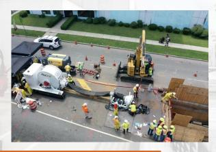
The Starline® Cured-In-Place (CIPL) lining application is a trenchless technology designed to recondition and renew existing metallic gas and pressure pipelines.
