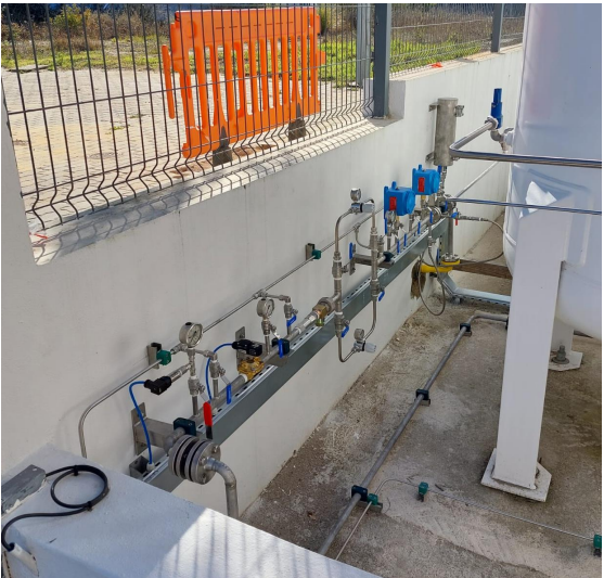
H2 pressure regulation and odorization at Gestene
