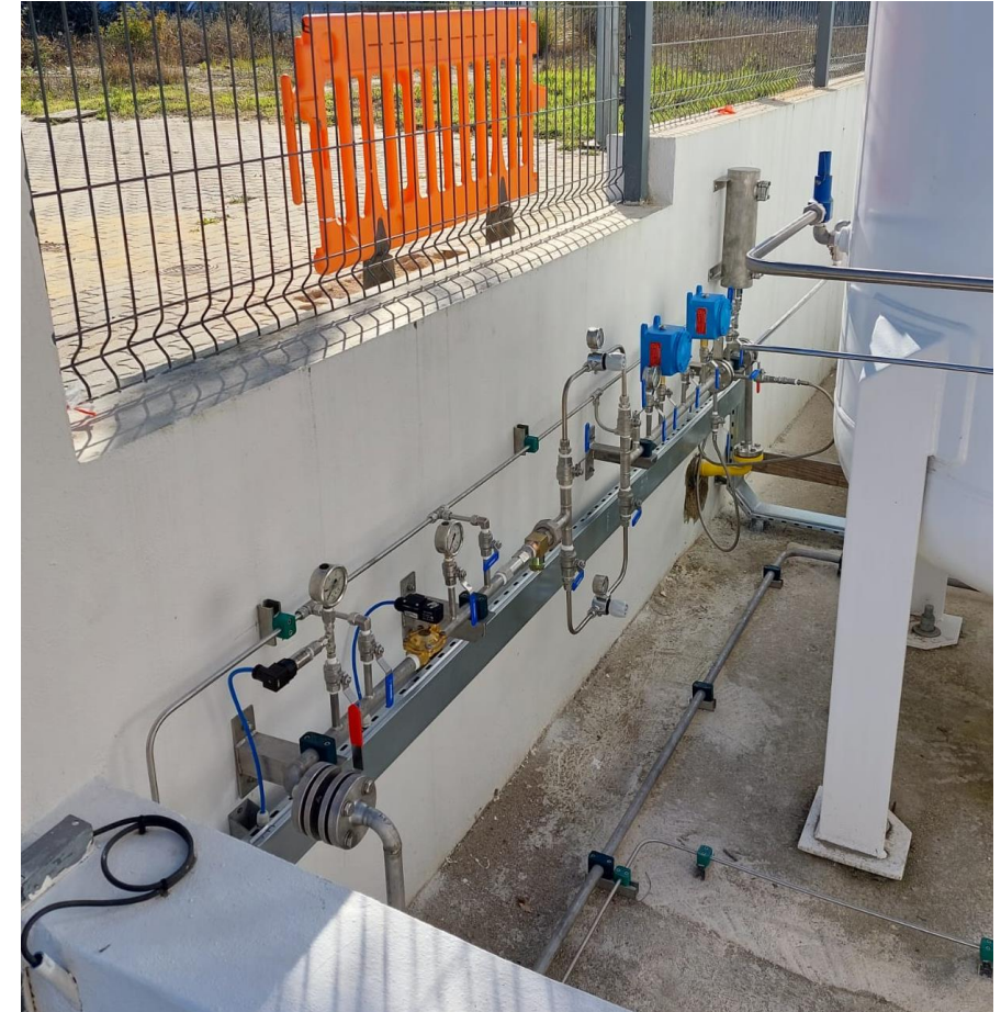
H2 pressure regulation and odorization at Gestene
