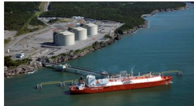
Canaport LNG. Photo courtesy of Repsol
