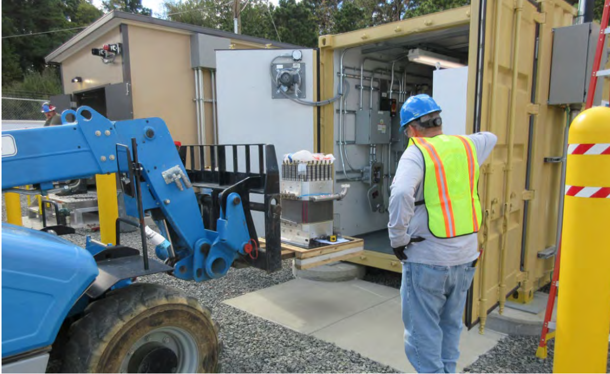
Electrolyzer Stack Installation
